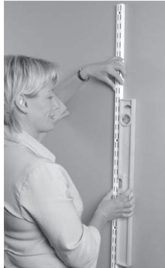
**Step 2** Check with a level that the wallband is hanging in vertical position.
