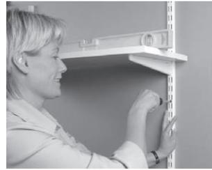
Install the second wallband. Use a shelf as a level to check that the wallband is placed in balance.
