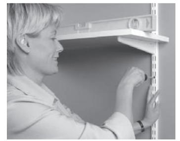
**Step 6** Place a shelf on the brackets and check with a level that brackets are in level. Drill holes and fix the wallband with screws.
