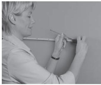
**Step 5** Prepare for the second wallband by measuring and mark the c/c-distance, not more than 900 mm between the wallbands. Place a bracket in the second wallband on the same height as the first one. Be sure of placing the wallbands parallel with one another and to place the both brackets in the same height.
